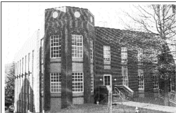
Binn-Merrill's new annex is the only section of the building which will be usable as the rest of the buildings is closed for renovations.
