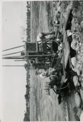
Drilling from barge in St. Lawrence River
