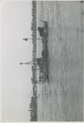
Drilling from barge in St. Lawrence River
