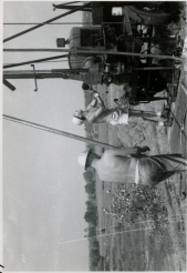
Lowering core barrel
