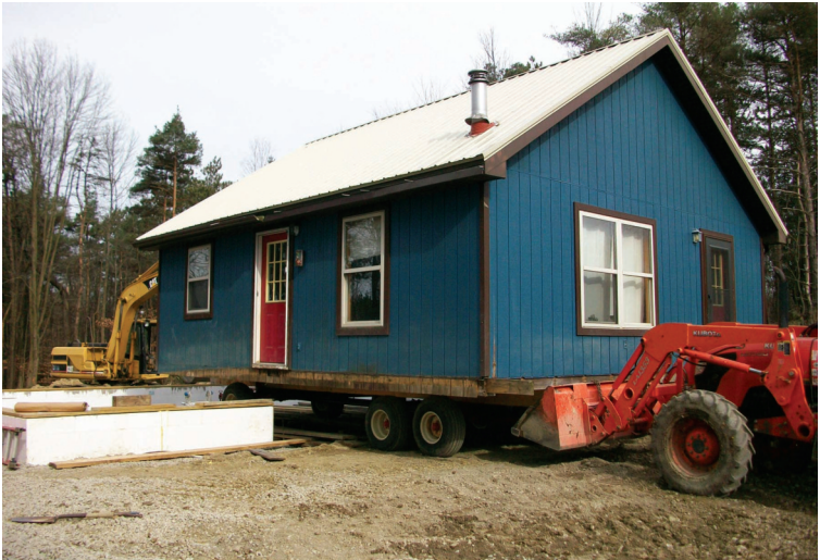
Positioning the house above its new foundation by pulling it with a front end loader and pushing it with a bulldozer.
